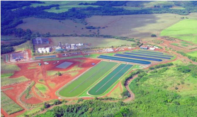
General Atomics, Kauai Facility, March 2012 | CO 2 is supplied from KIUC power plant (Photo courtesy of General Atomics)
